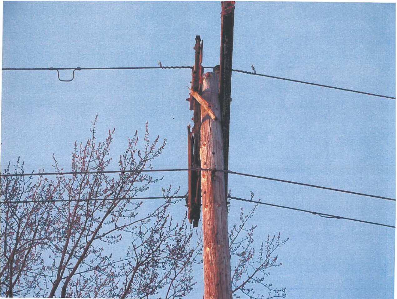
Photo B 3-19 Taken April 19, 2014 after contact was made. Taken from below Pole 24 of W185. Looking northerly, phase 1 conductor and insulator are near the base of the wooden pole. Based on angle of camera the upper wire is phase 2 conductor, the middle wire is neutral and the lowest wire is the phase 3 conductor. Photo provided by Public Service of New Hampshire
