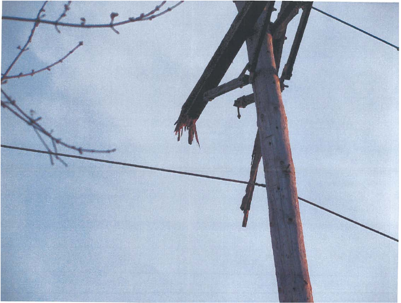
Photo B 3-18 Taken April 19, 2014 after contact was made. Eastern side of cross arm for Pole 24 of W185. Phase 1 conductor and insulator are near the base of the wooden pole. Lower wire is the neutral wire. Upper wire is the phase 2 conductor. Photo provided by Public Service of New Hampshire
