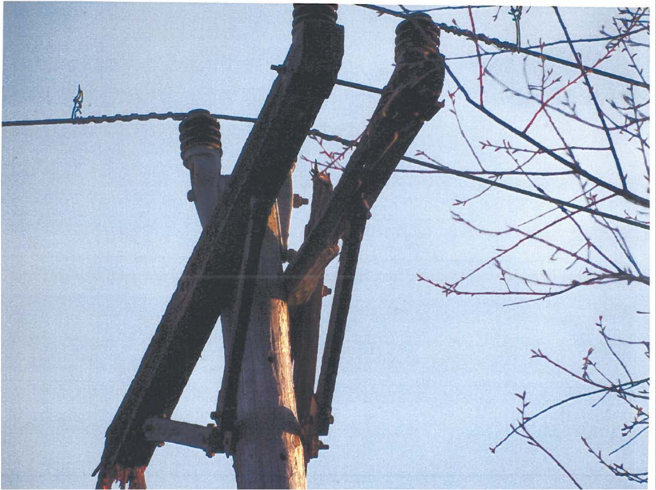
Photo B 3-16 Taken April 19, 2014 after contact was made. Collapse and failure of cross arm for Pole 24 of W185. Phase 2 and 3 conductors and insulators are intact. Photo provided by Public Service of New Hampshire
