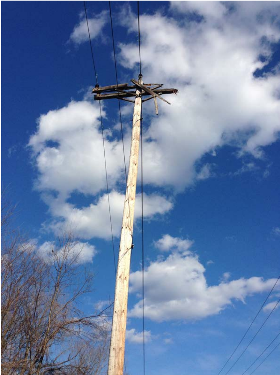
Photo B 2-4 This photo taken on the day of the electrical contact after the Fire Marshal arrived shows the W185 phase 1 conductor is missing from the double crossarm (attached to both sides of poles) that is completely broken and rotted. The conductor and supporting insulator is missing from the photo as it laying near the ground (see Photo B 2-5). Photo courtesy of NH State Fire Marshal's Office taken April 19 2014
