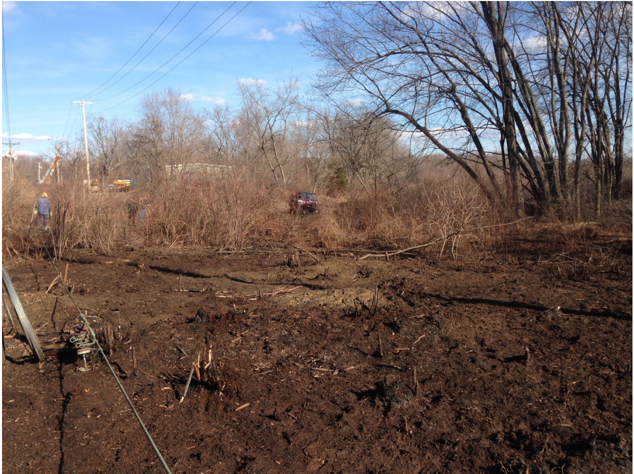
Photo B 2-7 Taken day of electrical contact April 19 2014. Looking easterly; displaying area of brushfire. Phase 1 conductor at the ground level. PSNH Work Crew had arrived on scene after contact occurred. Boom Truck is background. Insulators are on ground at base of Pole 24 of W185. Circuit W 15 is shown with all 3 phases intact. Photo courtesy of NH State Fire Marshal's Office
